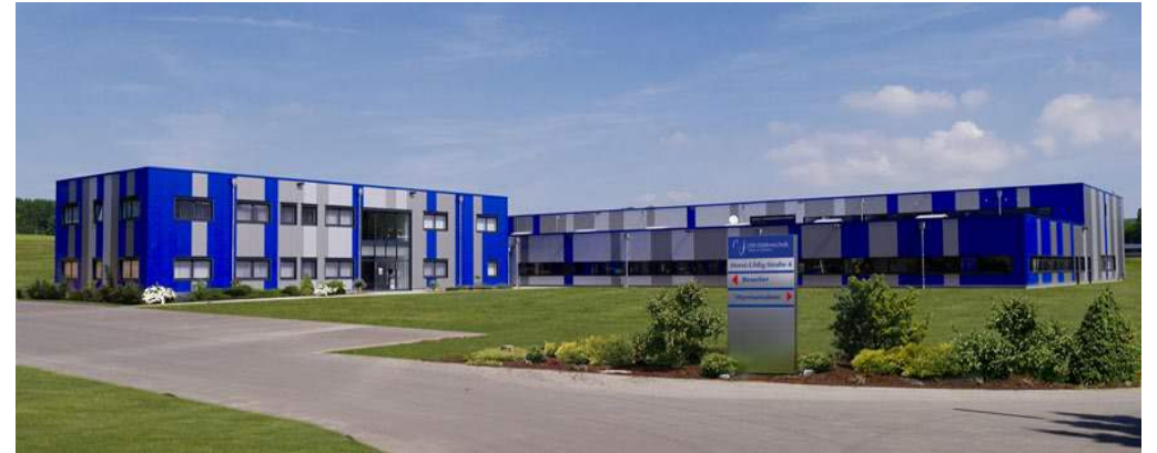
Schottel Factory-Laudert Germany
