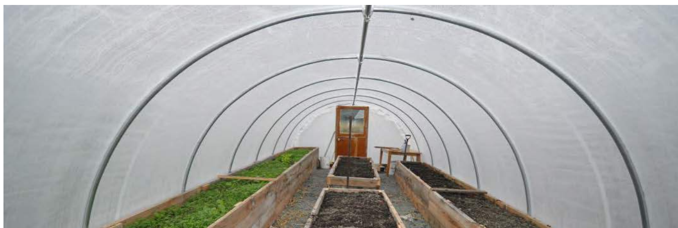
Newly constructed high tunnel in Haines.
