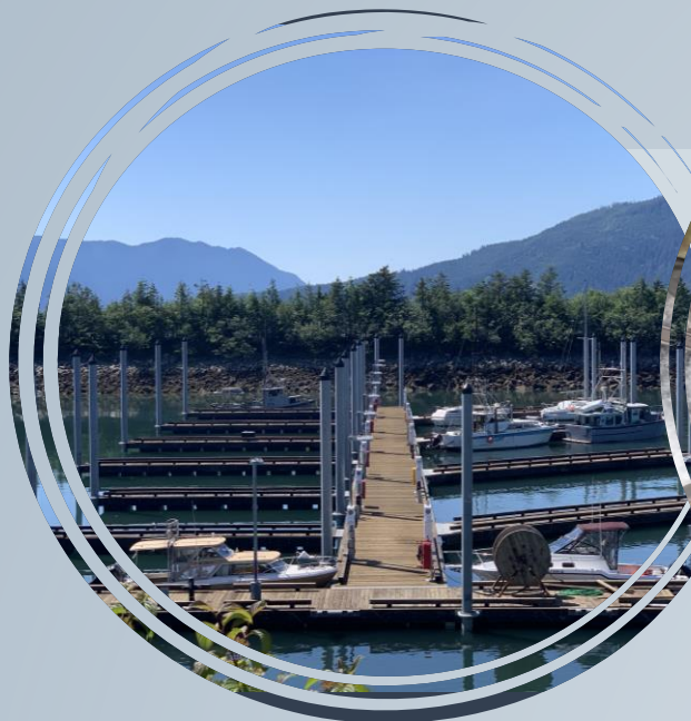
Steel anchor piles and mainwalks
