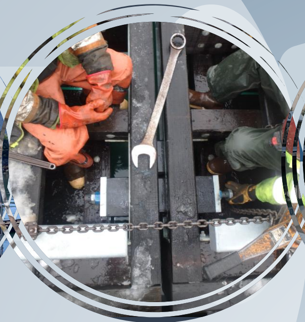
Float hinge connection shear block
